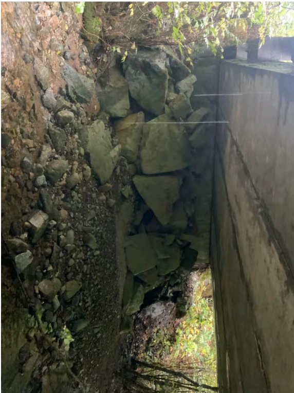
Right Bank Abutment when facing downstream
