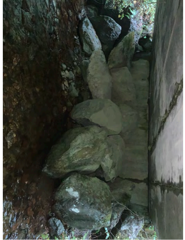
Left Bank Abutment when facing downstream
